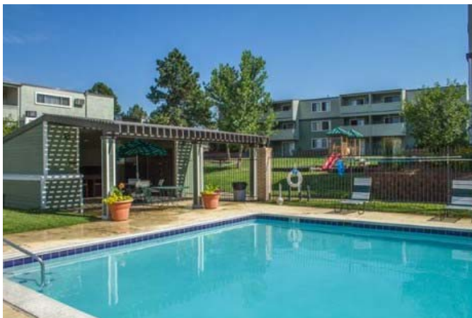
The company plans to improve the property and upgrade the general common areas and unit interiors.
